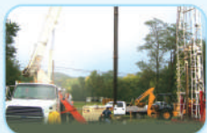
Deep Tube Well Construction
