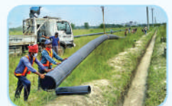
Water Supply Line Construction
