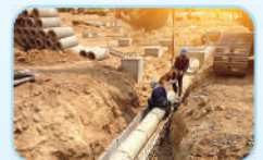
Drainage & Sewage Line Construction
